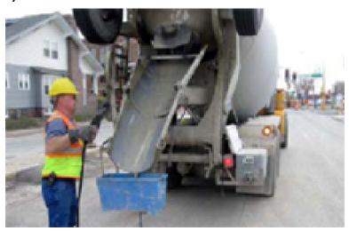
If there is very little concrete being used on site and the only washout required is the concrete chute then devices capable of containing all concrete liquids and solids can be used.
