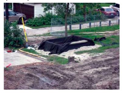
A berm trap system may consist of raised walls constructed from wood, straw bales, compost filter logs, sand bags, soil, lined concrete barriers, or any suitable strength materials to contain concrete washout liquids and solids until evaporation, curing, or extraction and final removal.
