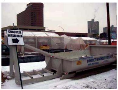
A skip washout system is capable of holding liquid and solid concrete washout materials until final treatment and disposal. Prevent commingling of other solid wastes with concrete washout materials.
