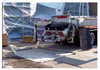
As a secondary containment method to avoid land and or water pollution, a Plastic drop sheet with weighed down edges can be used. This method is especially useful at connectors of the concrete pumper or under the chute of the concrete truck.
