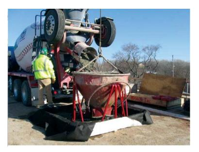
A rinse bucket separates concrete aggregate from washout water, and needs to be cleared of waste each day.
