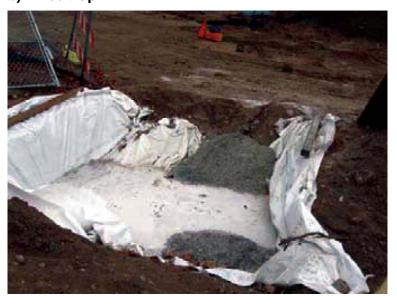
A lined trap system is excavated in an area with storm water overflow protection consisting of impervious plastic sheeting. The goal is to retain the liquids.
