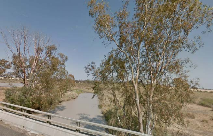
Photograph 12: Halls Creek – western side showing instream pools
