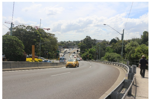
View from Bexley Road overbridge to Wolli Creek
