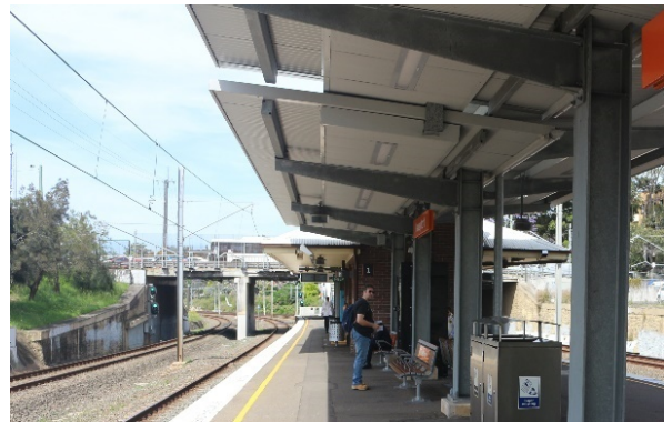
Heritage station platform building and overbridge
