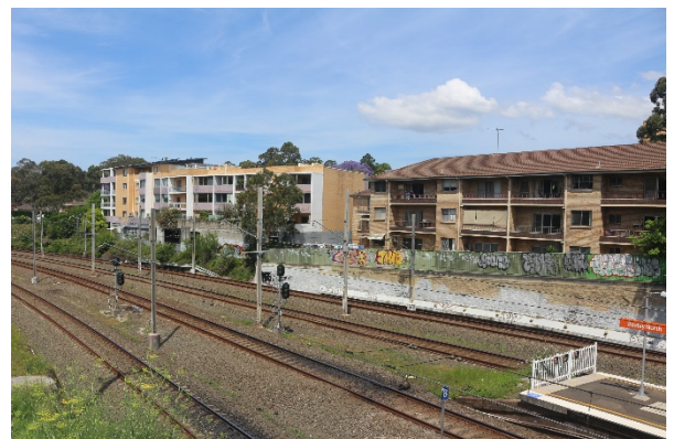
Residential apartment blocks in Slade Street, overlooking the rail corridor
