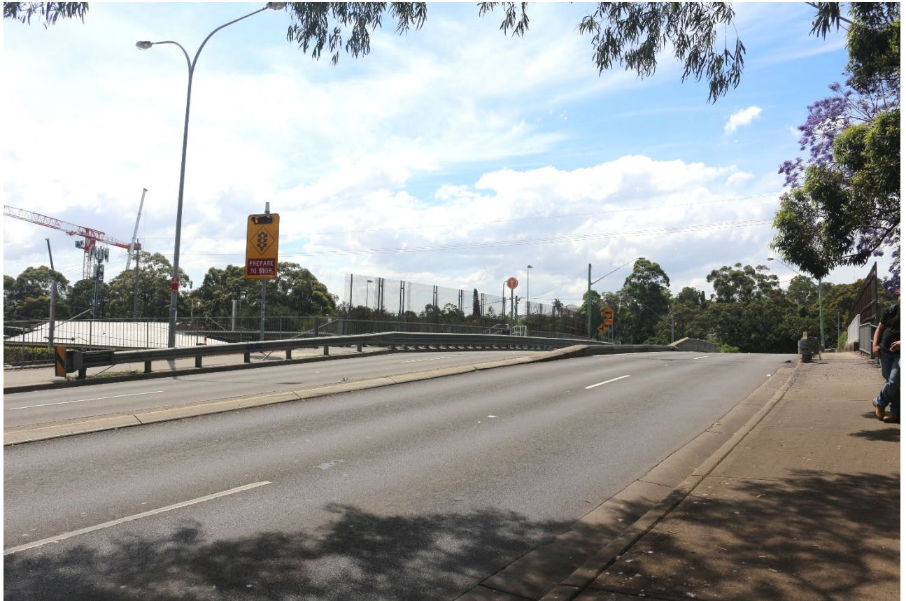
Figure 7-3 Viewpoint 1: View north west from eastern side of Bexley Road overbridge – existing view
