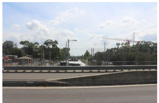
View west over station from Bexley Road overbridge
