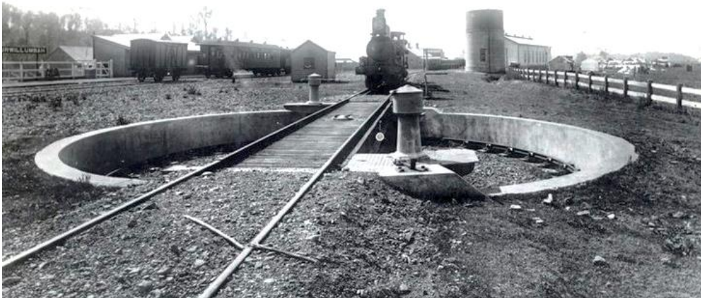
Figure 22. Murwillumbah railway turntable in 1904, showing the original 40ft turntable arrangement. This turntable, like Byron Bay, was replaced with a larger type in the early twentieth century. (Source: Tweed Library: MUS2015.60).
