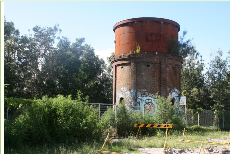
Figure 40. The Water Tower, seen from Butler Street.
