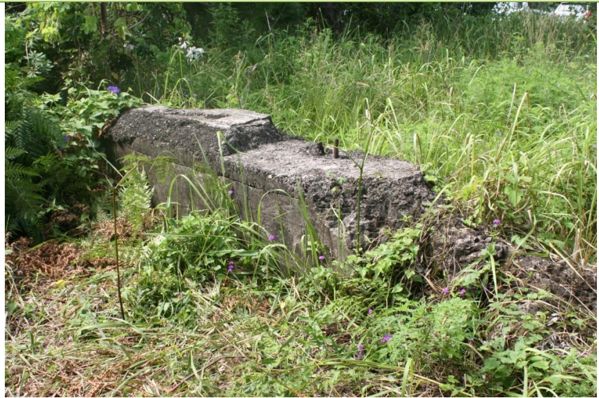
Figure 53. The northern concrete pier is largely buried in the ground.
