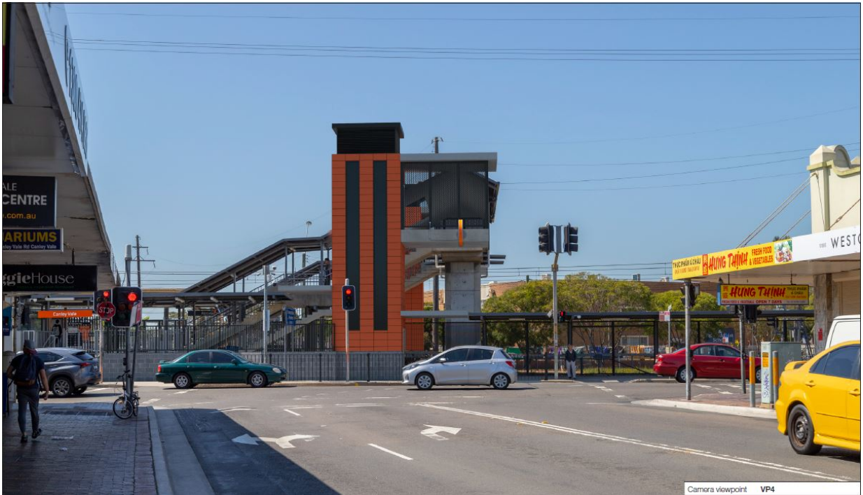
Figure 19 View from Canley Vale Road (west of the station) – Future View (indicative only, subject to detailed design)
