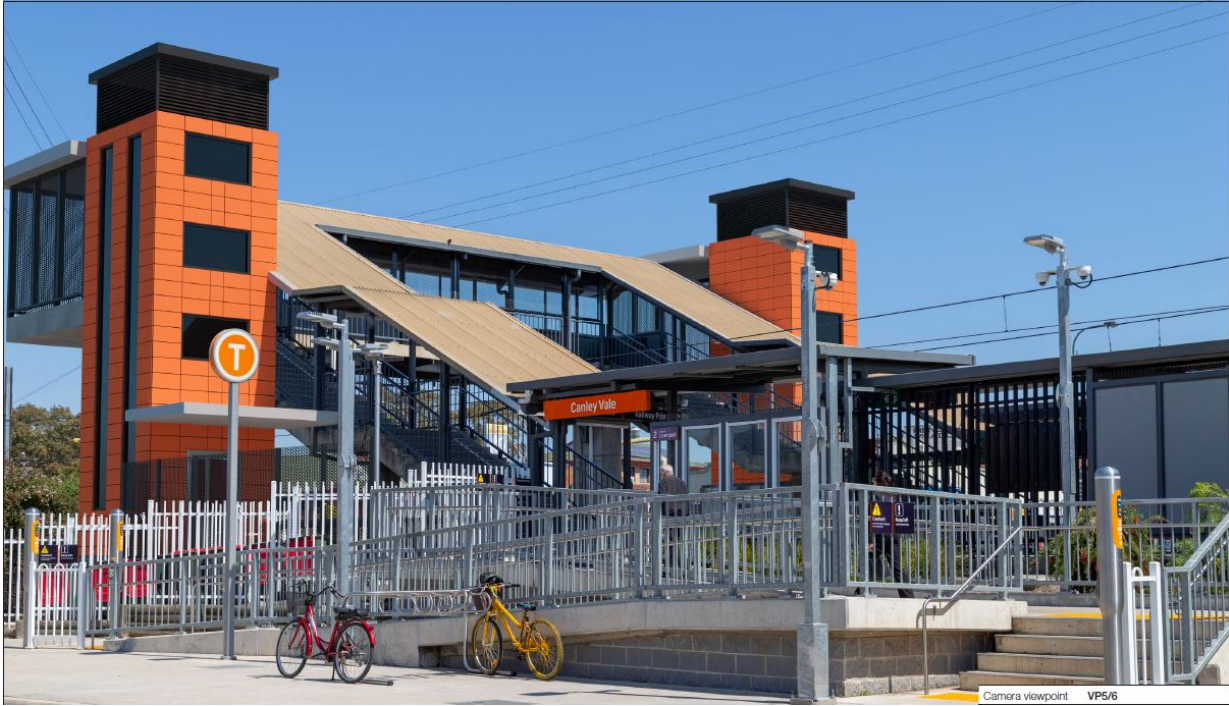
Figure 21 View from First Avenue / Carcoola Street intersection (east of the station) – Future View (indicative only, subject to detailed design)
