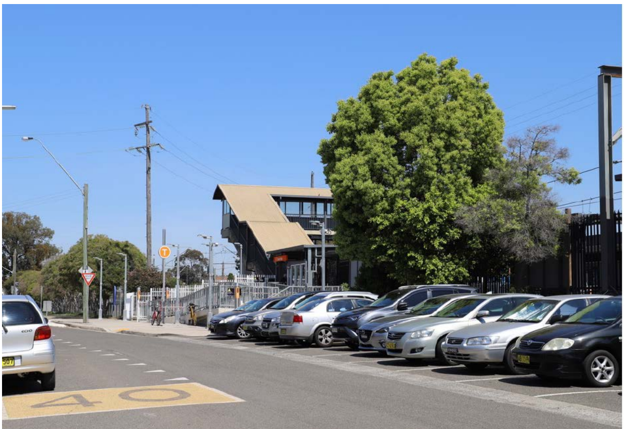
Figure 7 Existing view of Canley Vale Station from First Avenue
