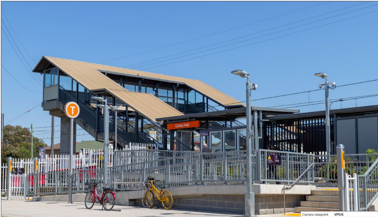
Figure 20 View from First Avenue / Carcoola Street intersection (east of the station) – Existing view
