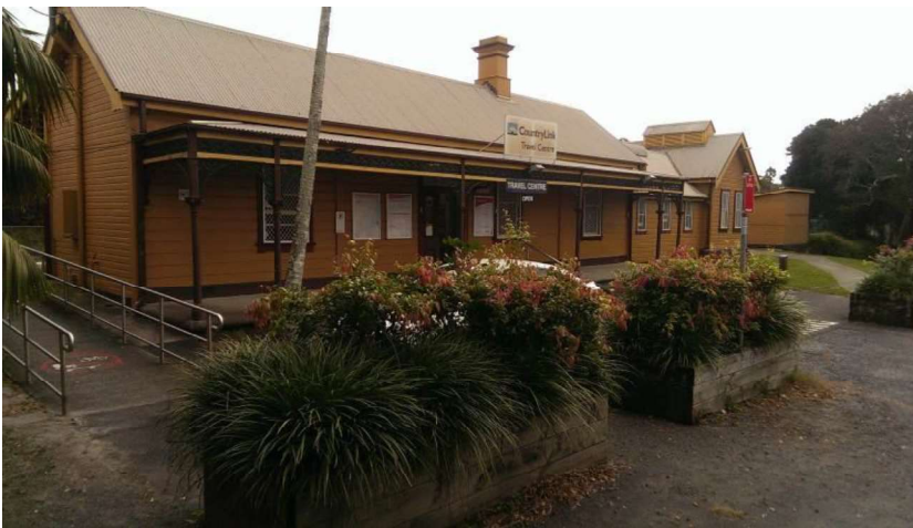
Photograph 4 The front elevation of the railway Station, looking north west, noting the planters.
