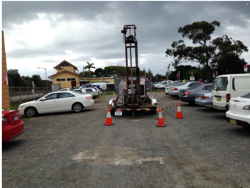
Plate 4: Drill rig with previous sample site in foreground
