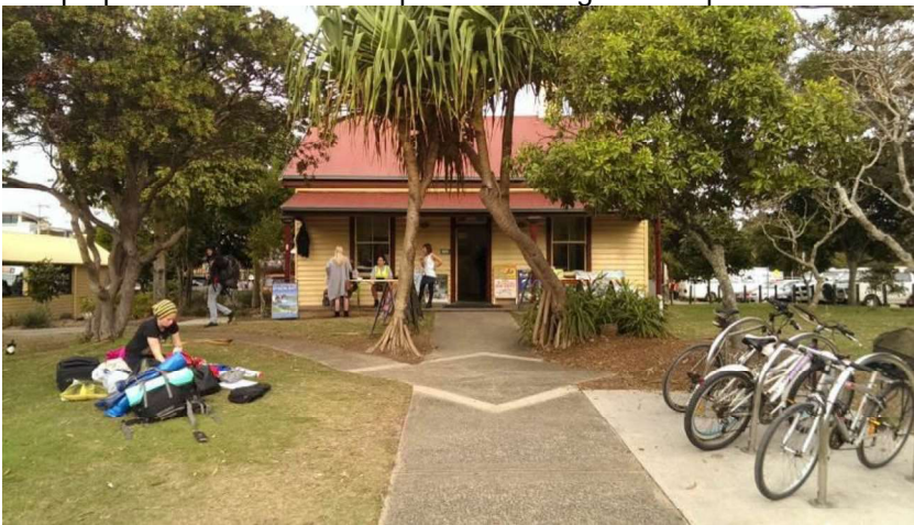
Photograph 7 The north elevation of the Station Master's cottage now Visitor information Centre
