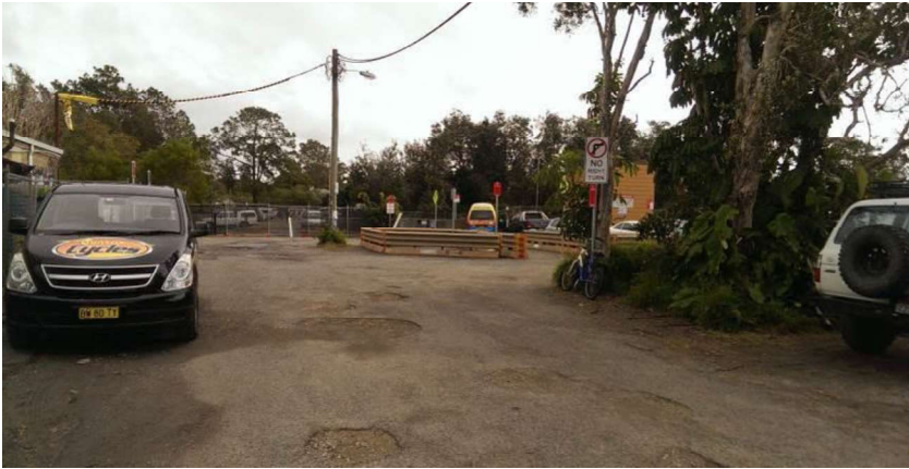
Photograph 21 View looking west down the Lane towards the level crossing. The Proposal removes the trees to the right and provides a raised island where the existing temporary barriers are located.
