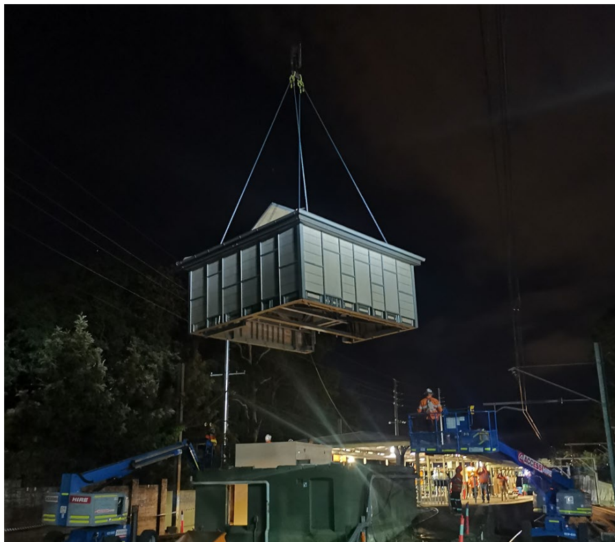
Image: installation of the lift shaft structure within the old booking office - during weekend work in March 2021.
