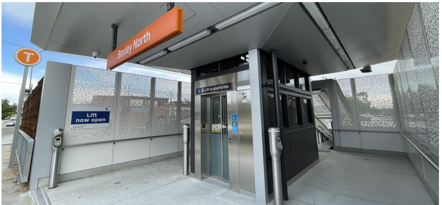
Above: The new lift at Bexley North Station is now open.
