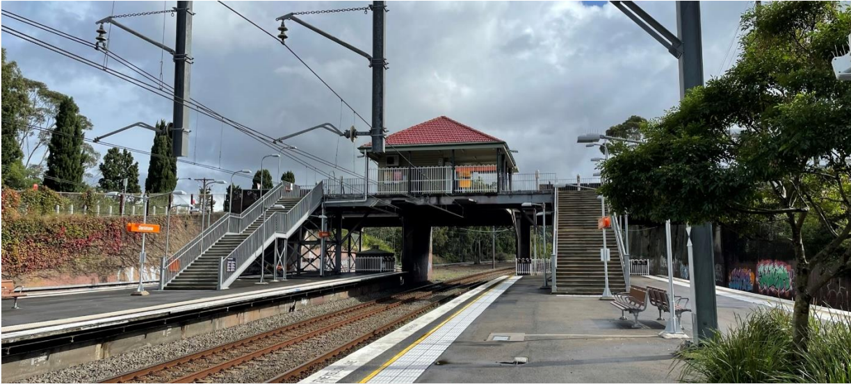
Figure 1-4 View towards station buildings and entrance from Platform 1/2
