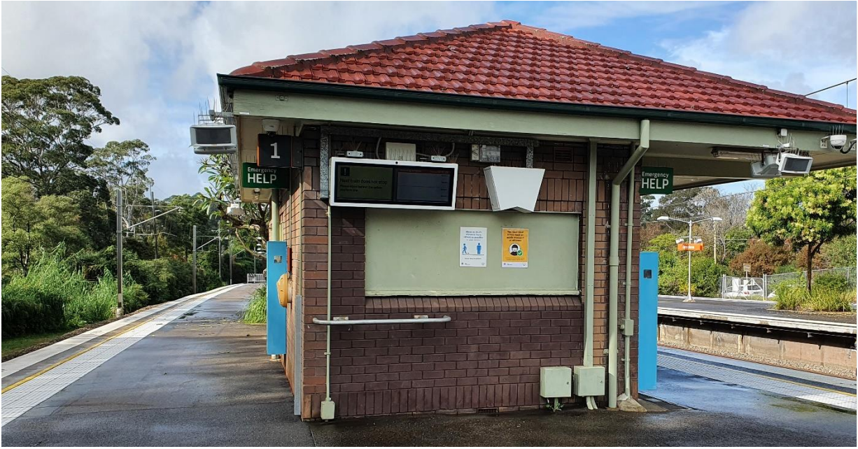
Figure 1-6 View of the existing platform building (existing toilets and store room) on Platform 1/2
