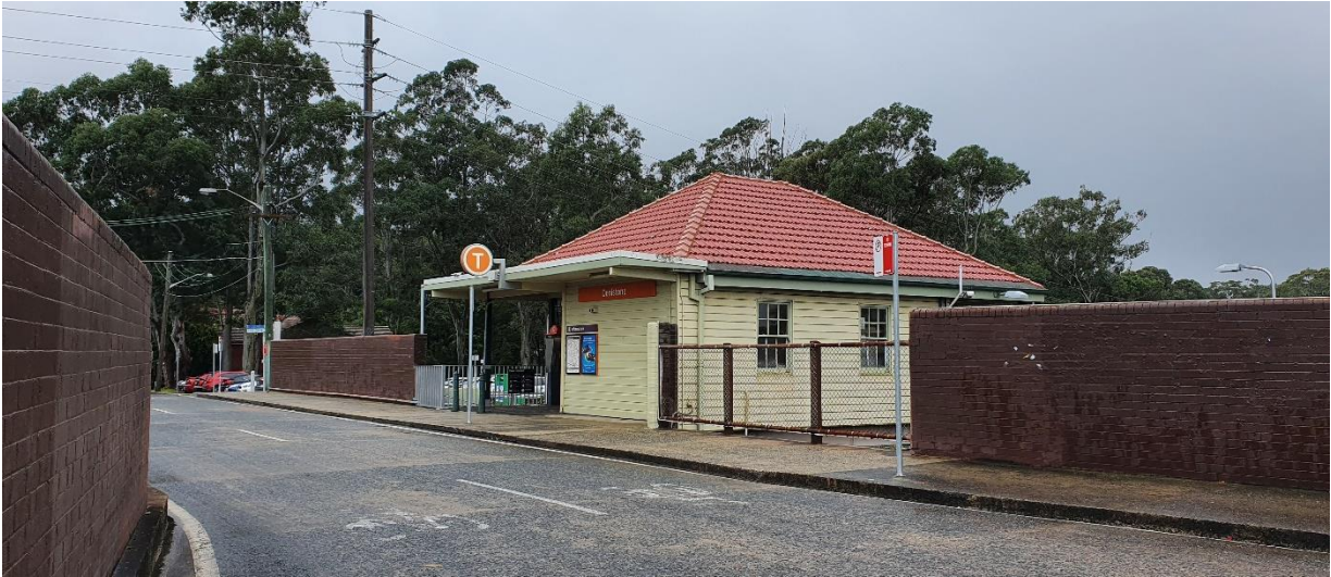
Figure 1-3 View of existing entrance from Gordon Crescent bridge
