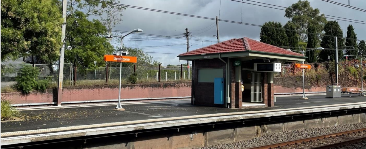
Figure 1-7 View of the existing waiting room on Platform 3/4
