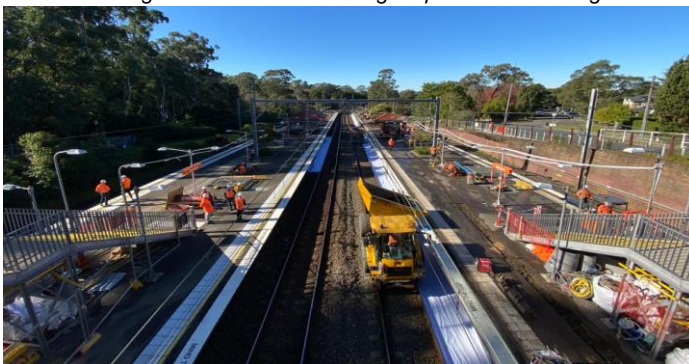
Work at Denistone Station in July
