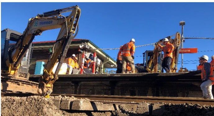
Building the under-track crossing for power and drainage
