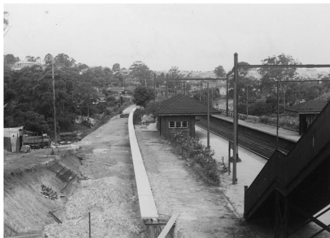
Denistone Station under construction. This picture shows the future proofing of the platforms to allow for new lines to be constructed. It also shows the plants and trees on the platform which was common for stations at the time.
