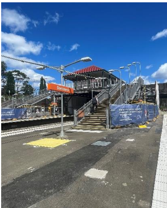
Denistone Station tidy up works – October 2022
