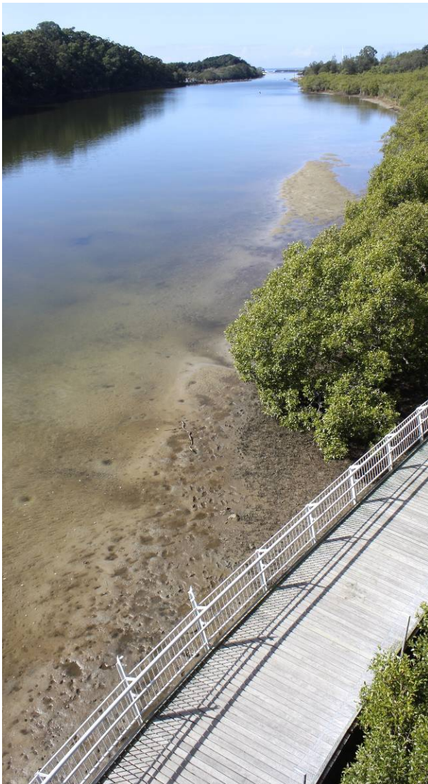
Brunswick River and boardwalk built as part of the upgrade
