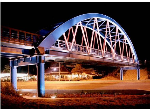
Coffs Harbour rail bridge over the Pacific Highway
