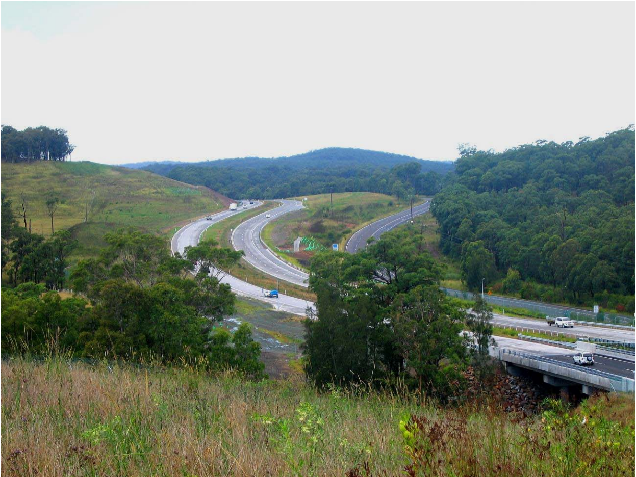
Karuah to Bulahdelah stage 1. A flowing responsive highway with flattened batters, a wide median and an alignment that skirts the hillsides.
