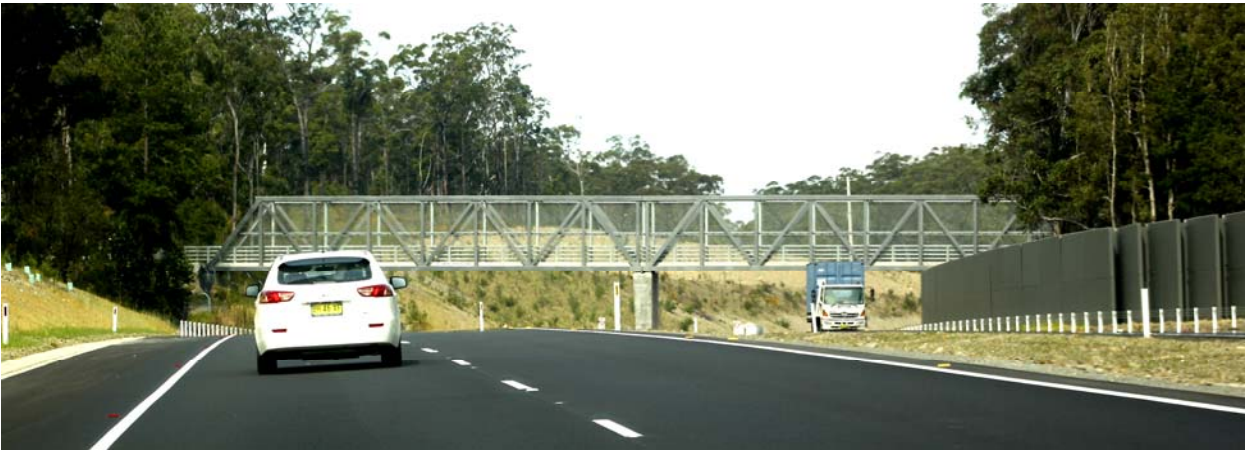
Truss bridge providing access to Alum Mountain and is a point of variety on the route
