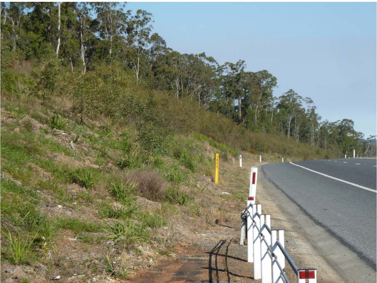
Cost effective revegetation of cutting slopes on the Glenugie upgrade through the spreading of existing forest soils with their natural seed banks.
