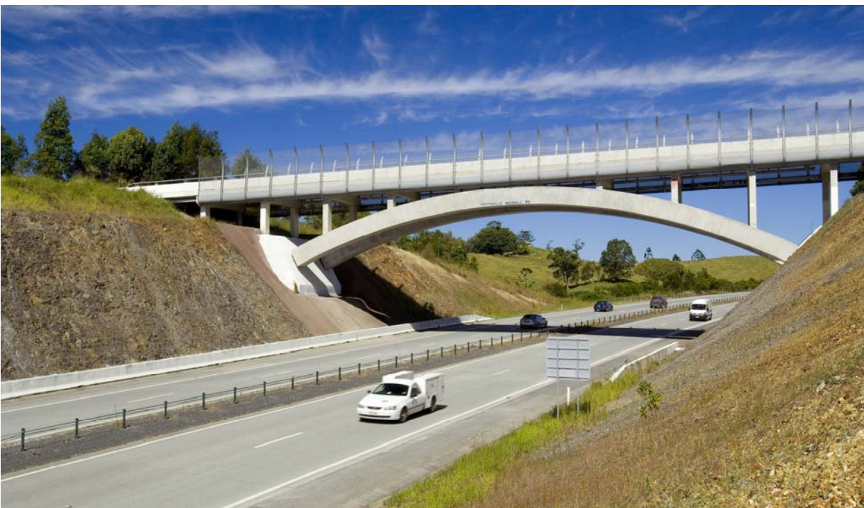
The opportunity to implement a sprung arch bridge was taken in this rock cutting. It provides an alternative interesting bridge design amongst the more prevalent standard overbridges.
