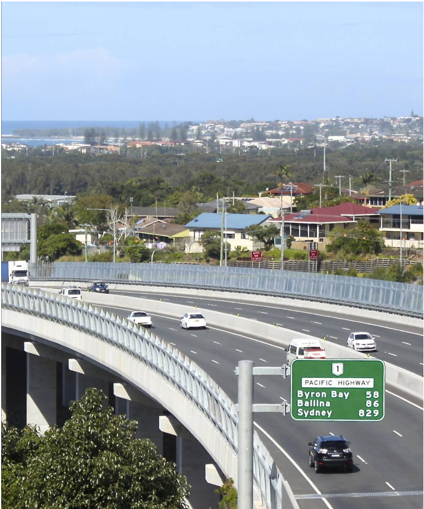
Banora Point upgrade is a landmark project marking the NSW Queensland border. The well designed viaduct with its views of the Pacific ocean, the deep cutting with feature lighting framing views to the gold coast, Wilson Park recreated on a landbridge and a new gateway to Tweed Heads.
