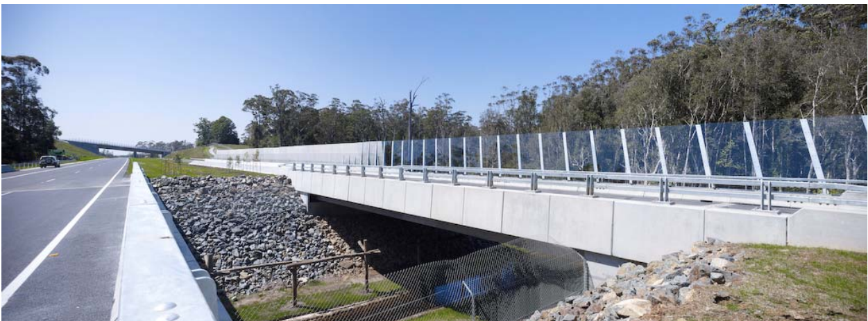
Clear acrylic walls on bridges marrying neatly with concrete walls on grade
