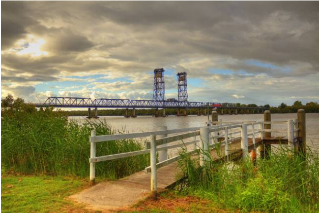
Bridge over the Clarence river at Harwood
