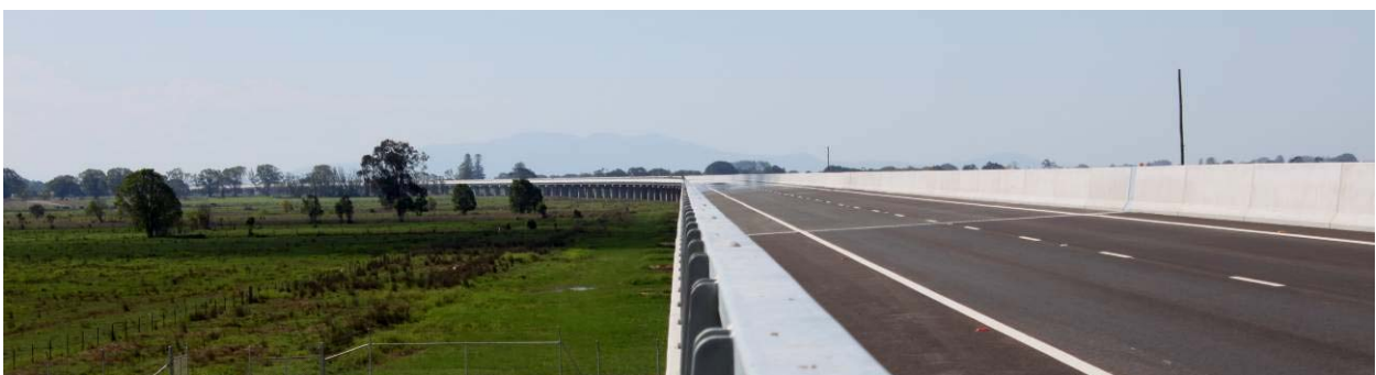
Kempsey bridge – the longest in Australia
