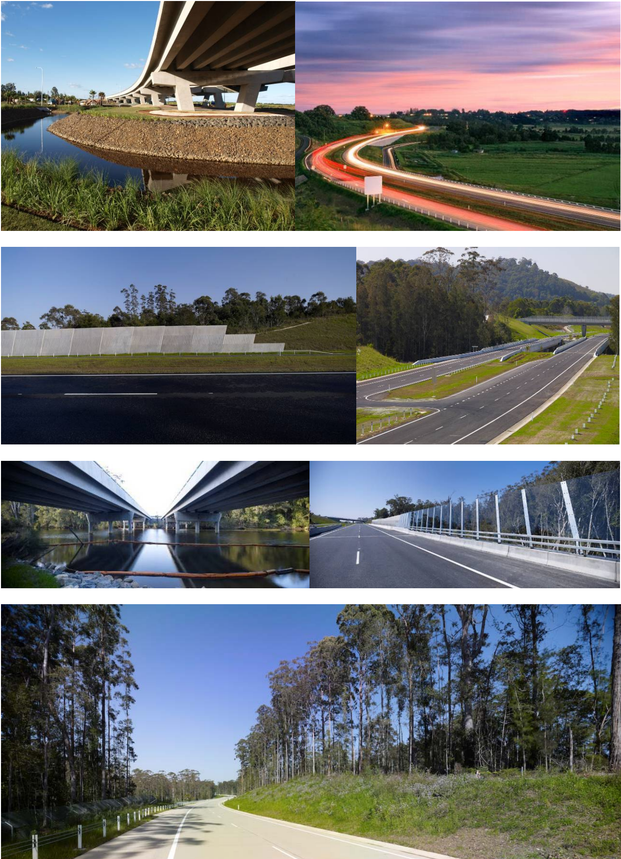
From top left to right: Ballina Bypass Teven interchange, Ballina Bypass alignment, Bonville upgrade noise wall, Bonville upgrade alignment and overbridge, bridges over Bonville Creek, clear noise walls over bridges, Pine Creek State Forest alignment.
