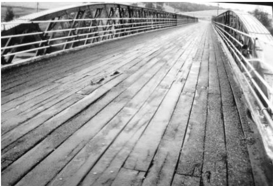
Typical timber deck on a lattice bridge at Forbes and the use of buckled plates
