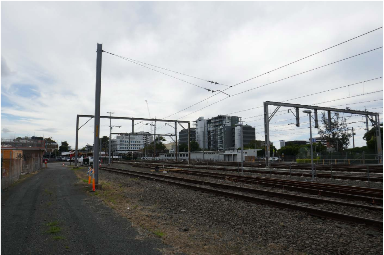
Figure 1-3 Wollongong Stabling Yard, looking north-east towards Wollongong CBD and Wollongong Station
