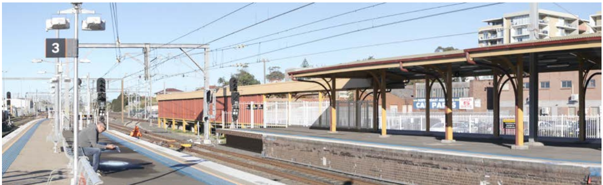
Figure 6-1 Existing and indicative future views of Platform 1 from Platform 2
