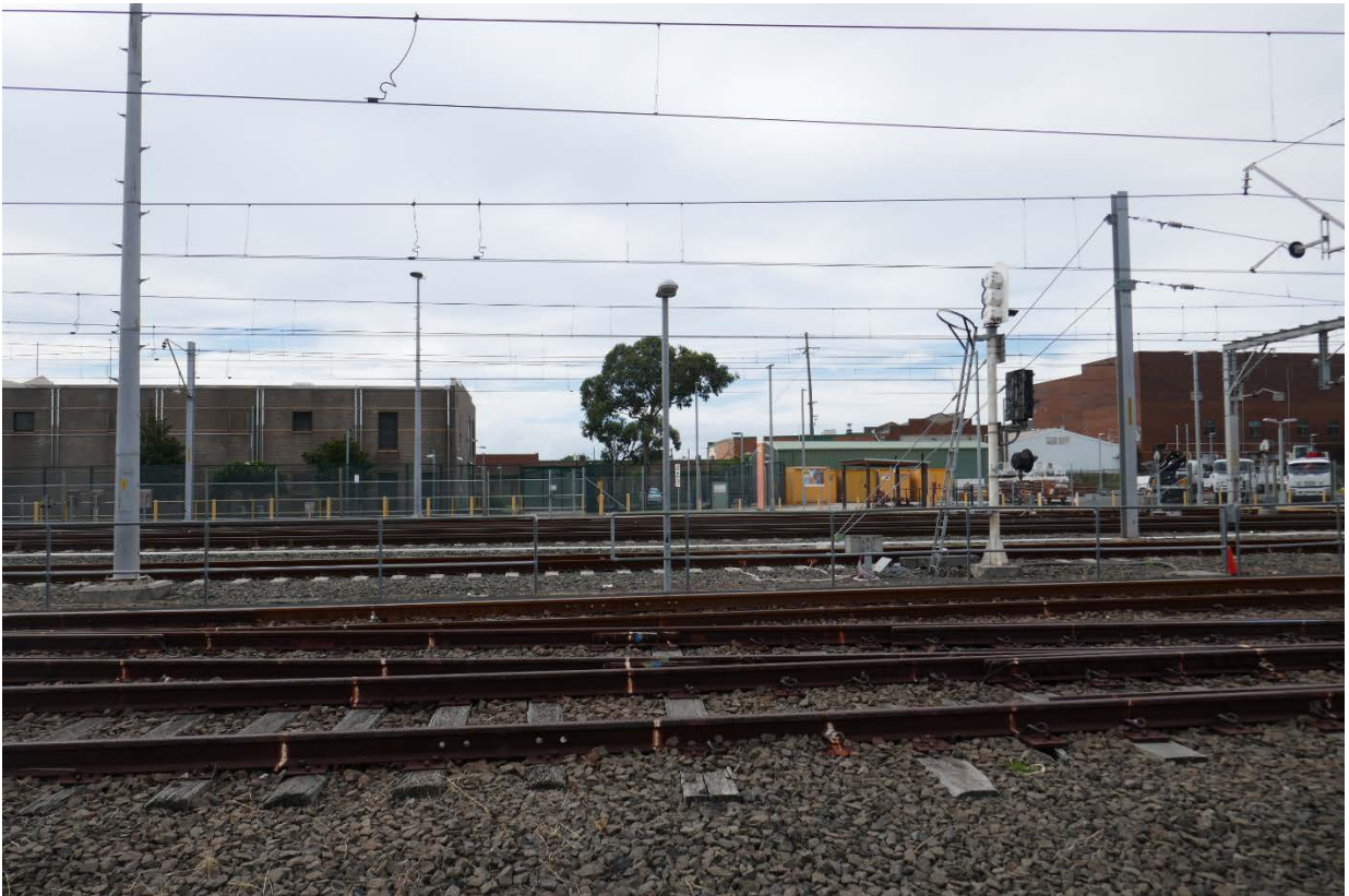
Figure 1-4 Wollongong Stabling Yard, looking east across the Up Yard towards the Down Yard
