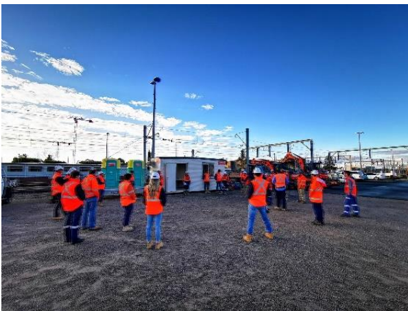
Members of the project team during an on-site briefing at Wollongong
