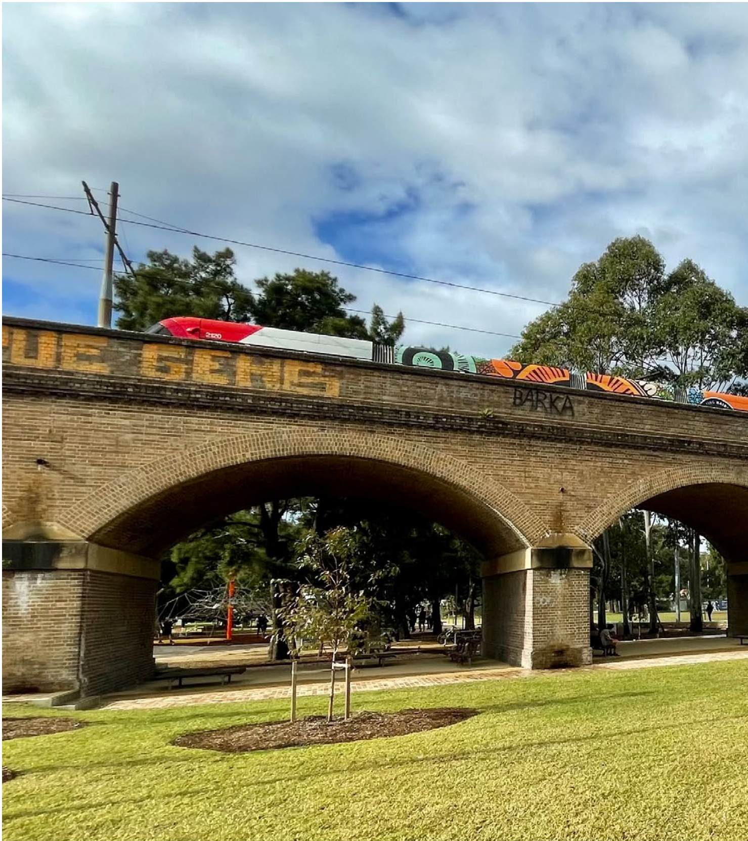
Light Rail viaduct Annandale — The multiple openings of the viaduct create a permeable structure for movement and views, good surveillance and no impediment to a good ground level space. In fact, interest is added to the spaces and views, if designed well. While this viaduct is old and a piece of important heritage, a similar effect can be achieved with more modern bridge viaducts.
