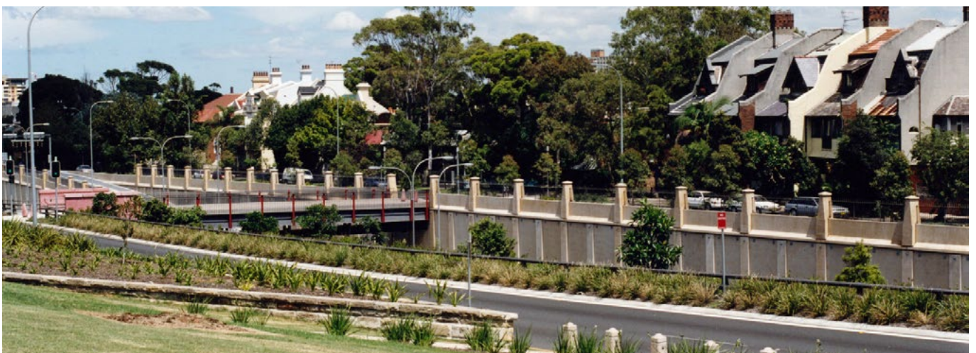
Eastern Distributor shortly after opening in 1999, illustrating the road alignment lowered and street level bridges connecting the local roads and footways to the adjacent park.
