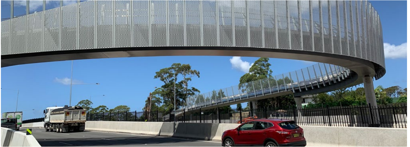
Pedestrian bridge utilising the falling grade of the road to provide a relatively flat grade crossing with views and good passive surveillance (Northern Beaches Hospital road upgrade)
