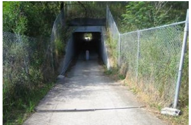
M2/Vimiera Road, Marsfield — The approach to this underpass is surrounded by dense vegetation, lacks a sense of space due to the fencing and portal design, and does not afford good surveillance from the surrounding area.
