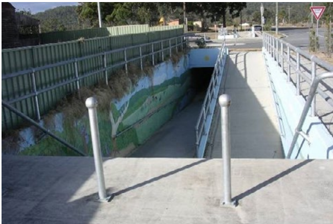
Coolongolook — This underpass is approximately 35 metres long and 2.4 metres wide. Having sunken approaches with no visibility through to street level it does not offer good passive surveillance nor a direct route.
