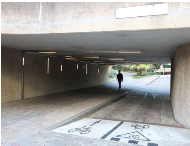
Retrofitted lighting at Kent Street, integrated into the ceiling and wall made from stainless steel with thick acrylic diffusers.
