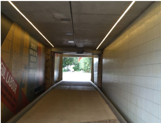
Strip lighting designed into the Lennox Bridge underpass, vandal resistant, constant light source and an attractive element complementing the space. The use of tiles provides a lighter more vandalism proof finish.
