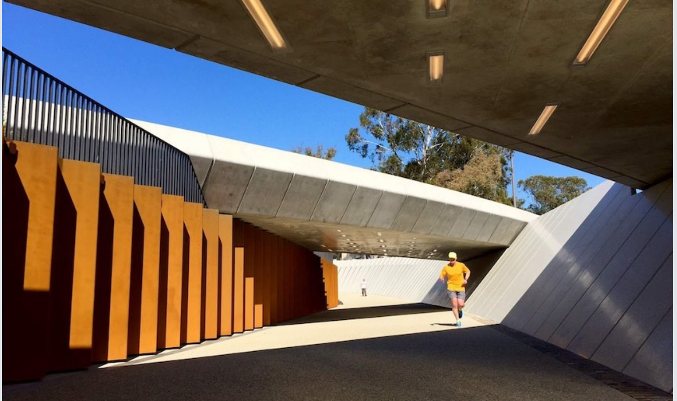
The Bowen Place Underpass, near Kings Avenue Bridge, took out a top award for infrastructure (ABC News: Mark Moore)
