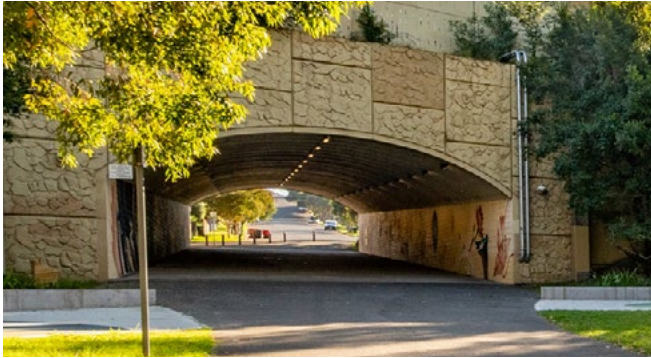
Underpass on the M5 East, Bexley. The trees around the portals improve the outcome and visually reconnect the two sides of the passageway.
