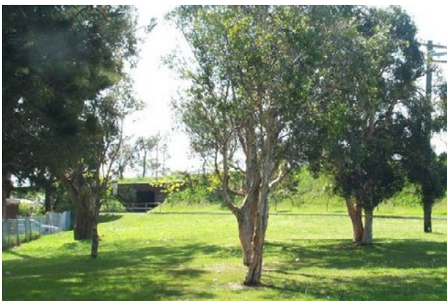
Gardeners Road, Sydney — This utilitarian underpass is located in an out of the way location with very little passive surveillance. The approach path is not in line with the underpass itself and visibility through the underpass is poor. At 2.4m metres wide and 45 metres long, it is too narrow.
