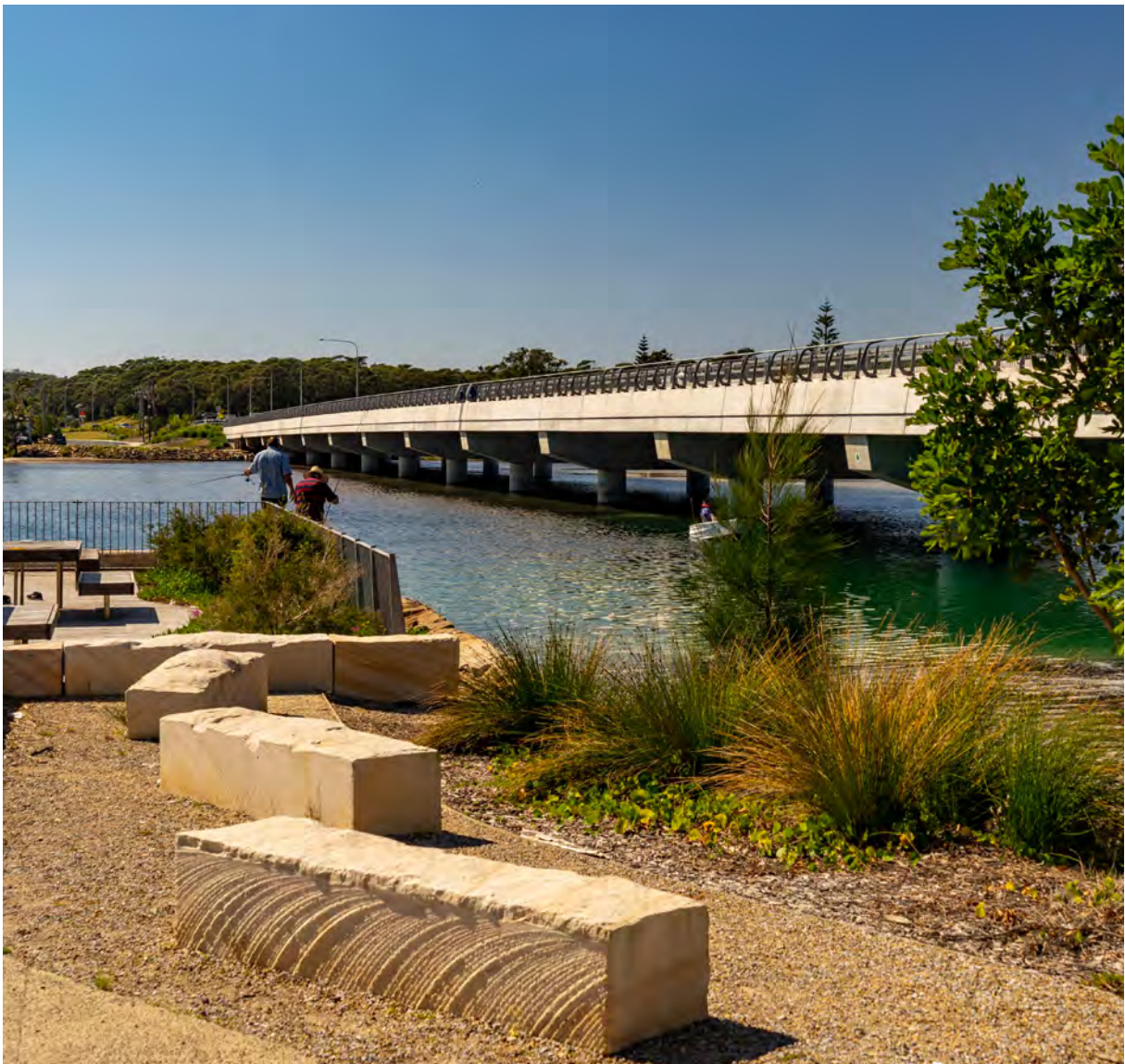
Burrill Lake reuse of old bridge abutment
