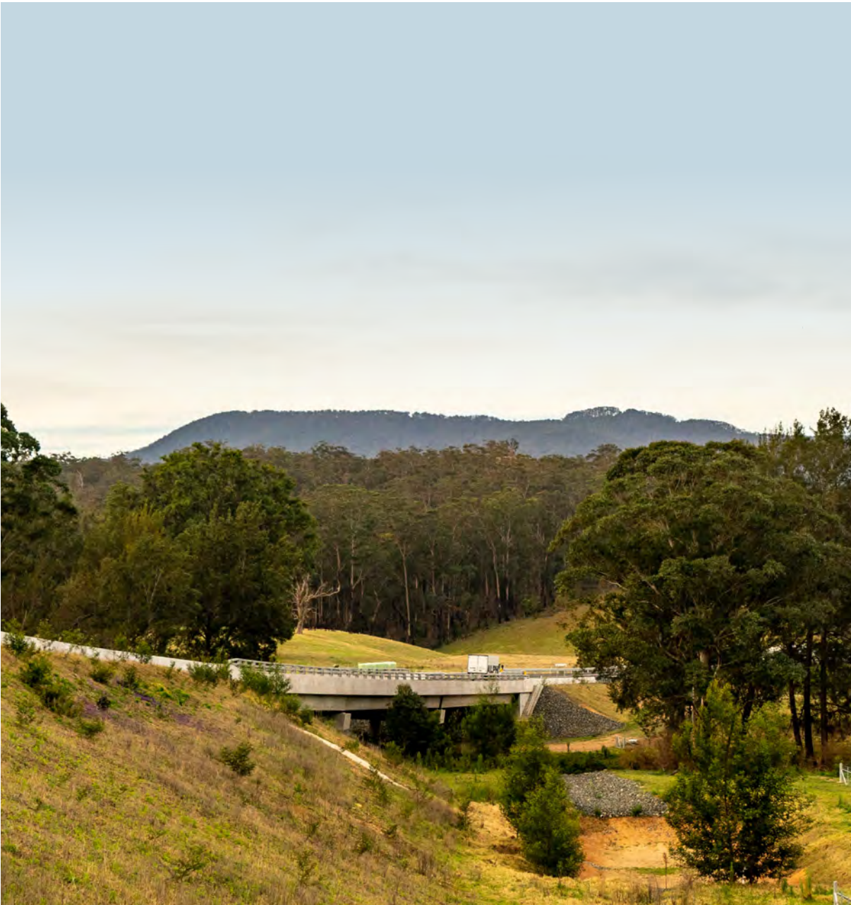
Embankment graded to 1 in 3
