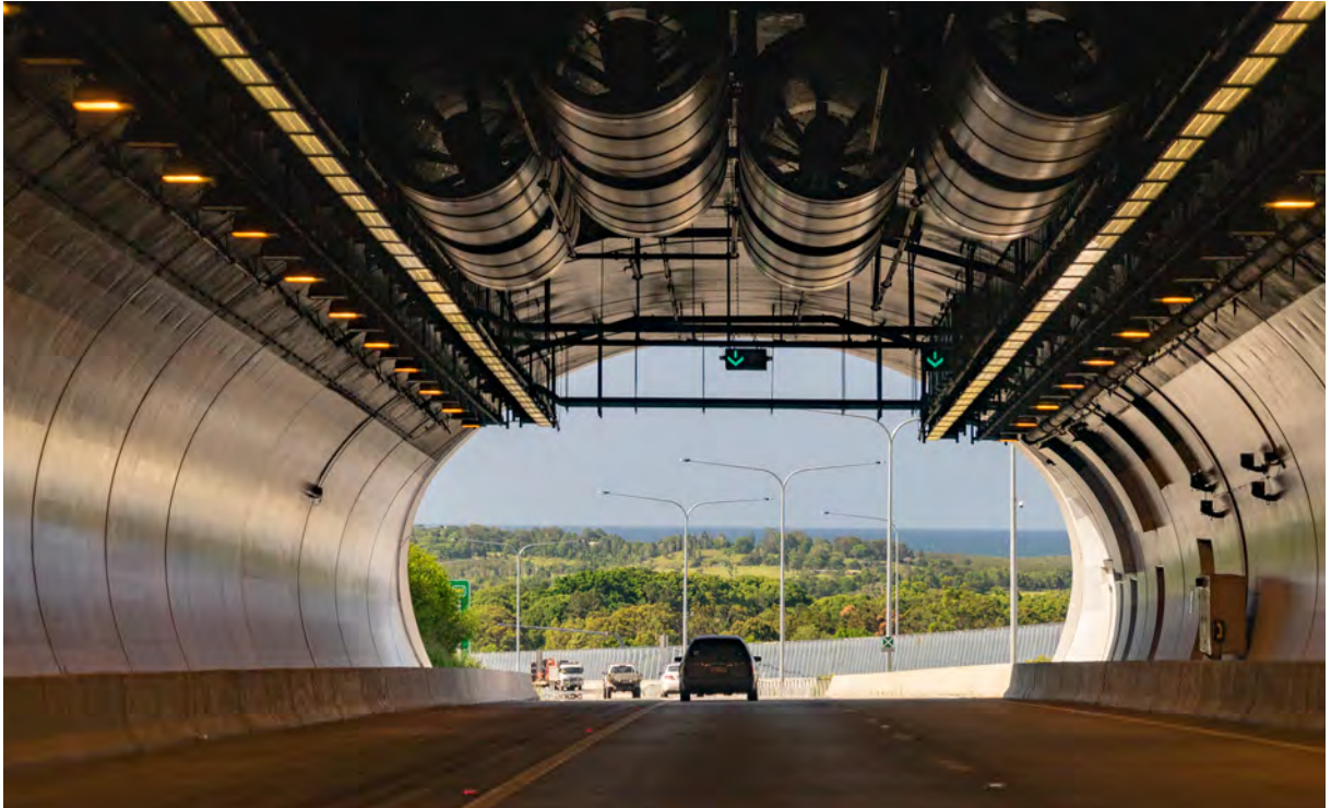
Tintenbar to Ewingsdale tunnel
