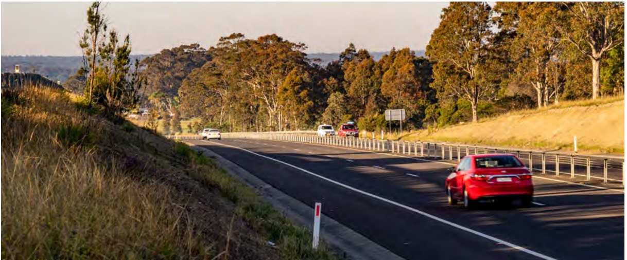
Use wire rope fencing where practical to allow the views of the landscape and a less 'walled' environment, which is in keeping with the south coast
