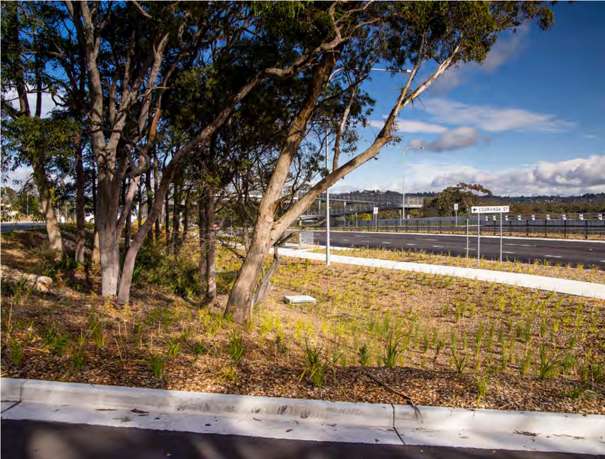
Use the landscape to capture clean and use water for plant growth (Bullaburra, Great Western Highway)
