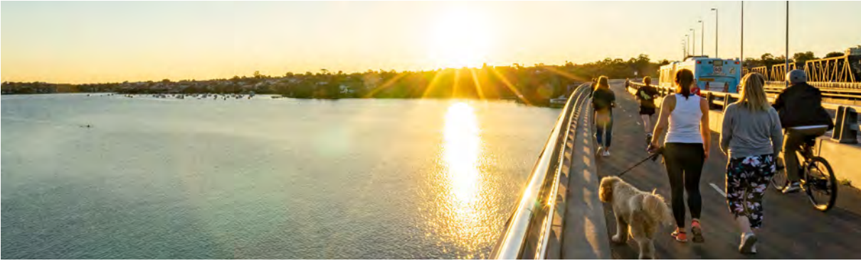
Burrill Lake Bridge above. Below The new Iron Cove bridge includes a 5m wide path which allows for regional connections as well as a waterside recreational loop.
