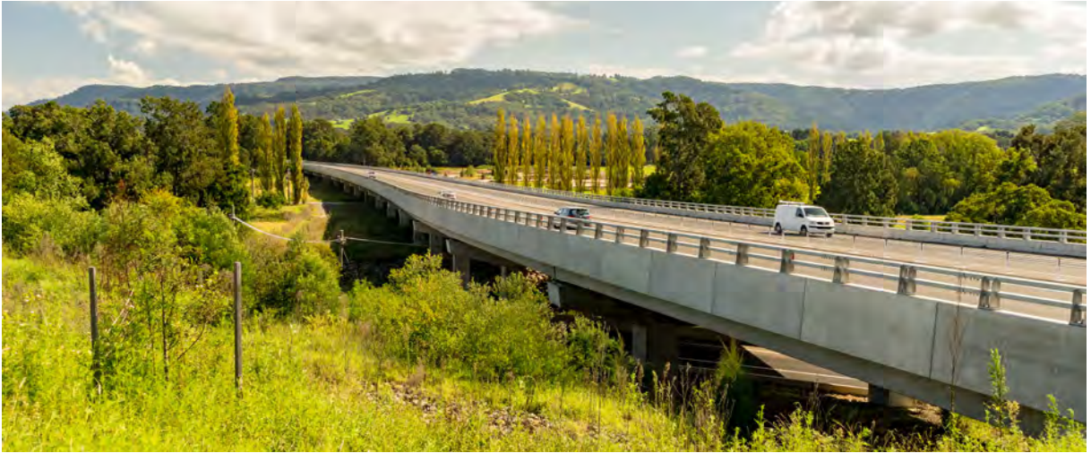
Two rail barrier on the viaduct passing Berry
