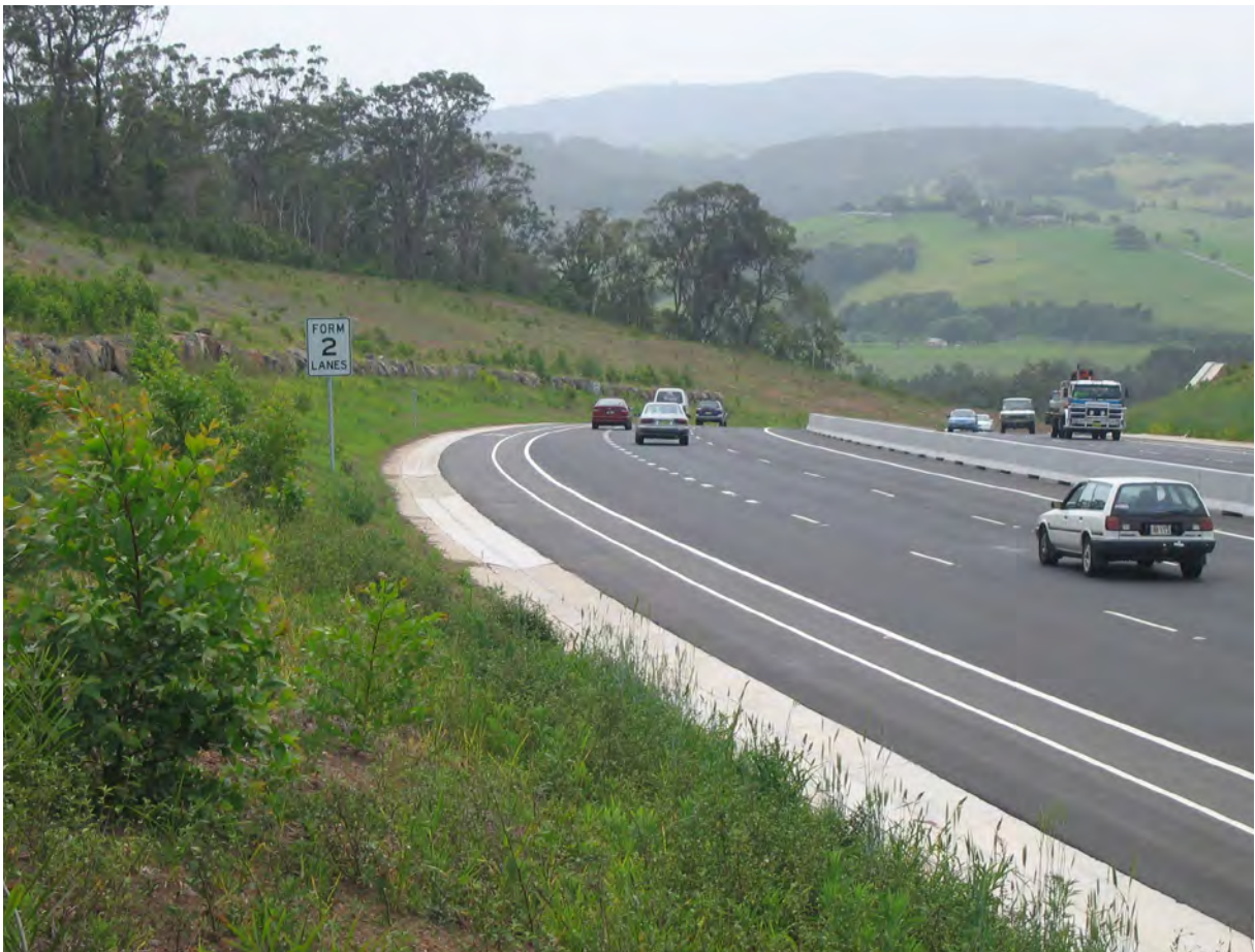
Shallow cutting on North Kiama bypass created using stone retaining walls
