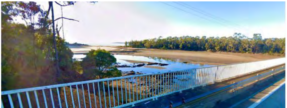
A classic south coast inlet and bridge crossing views of the water and a bushland fringe.
