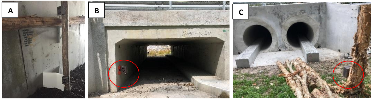
Plate 2: Typical underpass camera set-up: box culvert within sections 1-2 (A); Wardell Road box culvert – camera at each end (B); Wardell Road twin-pipe – camera at each end (C).
