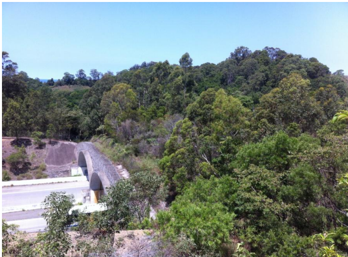
Site five, the fauna bridge at Taggets Hill
