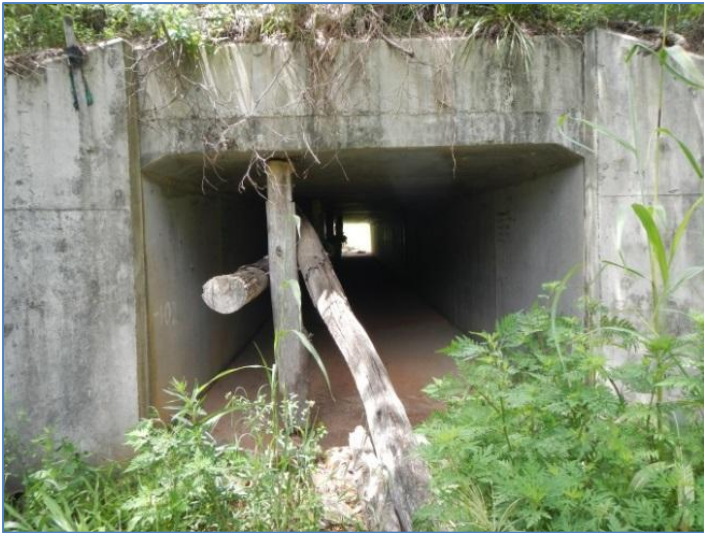
Site one, the culvert south of Eviron Road
