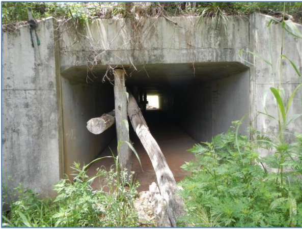
Site 1: Culvert south of Eviron Rd
